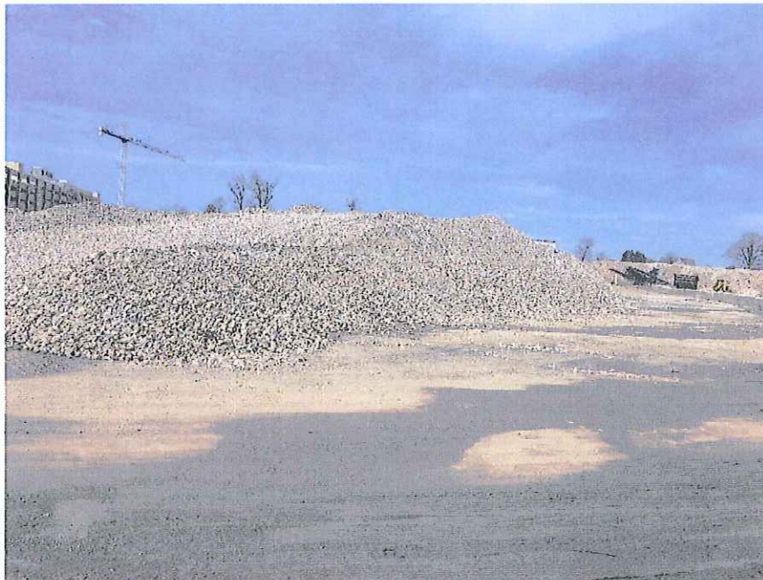
Crushed Concrete pile out front
