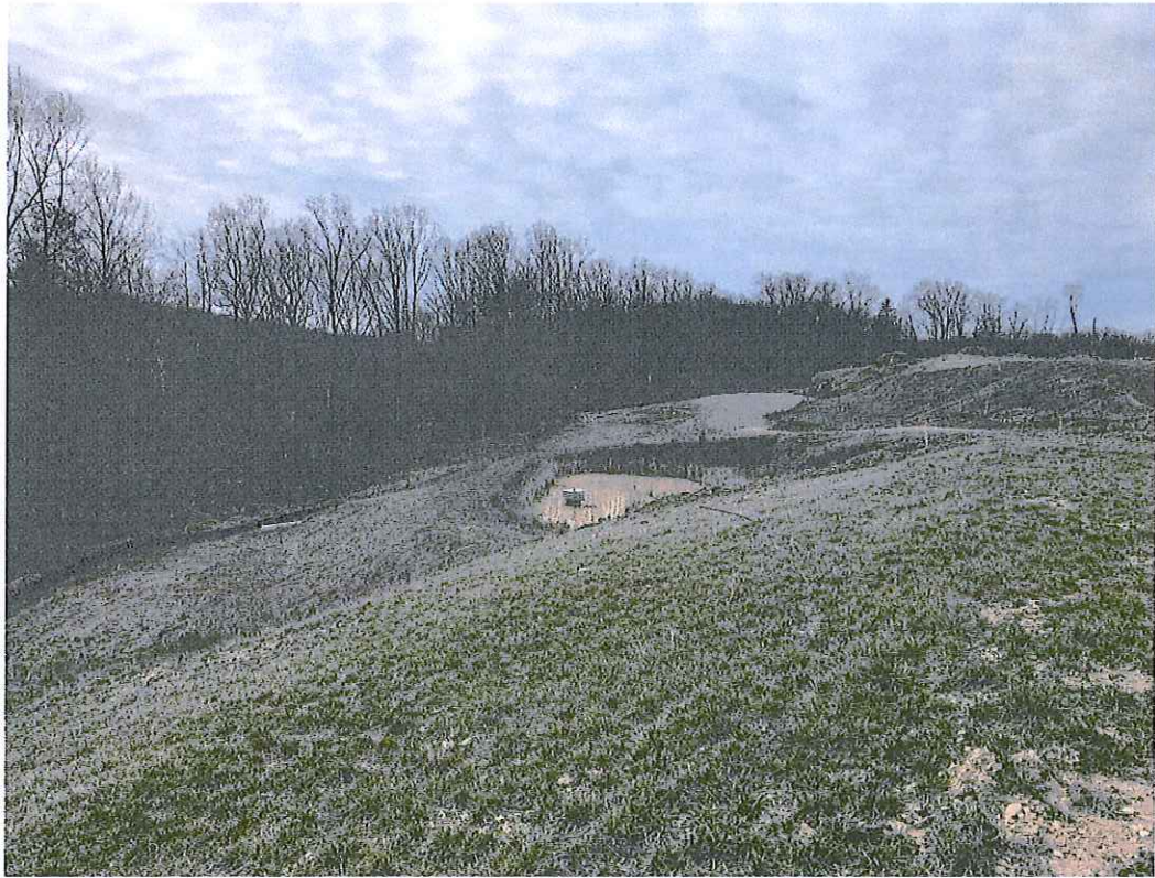
Earth work south side of FDA Boulevard
