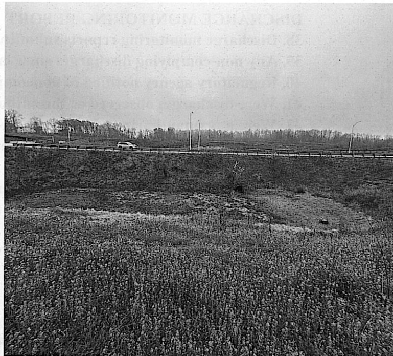
Figure 3: Sediment Trap along FDA Blvd.
