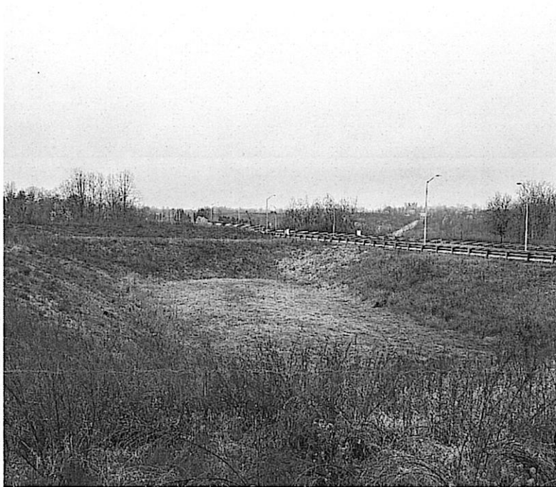
Figure 14: Sediment trap south side of FDA Blvd.
